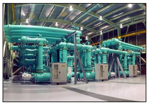
Figure 8.3: Gas insulated Substation (*Source: <u>http://kiran111.hubpages.com/hub/Gas-Insulated-Substation</u> 24-06-2013)*
