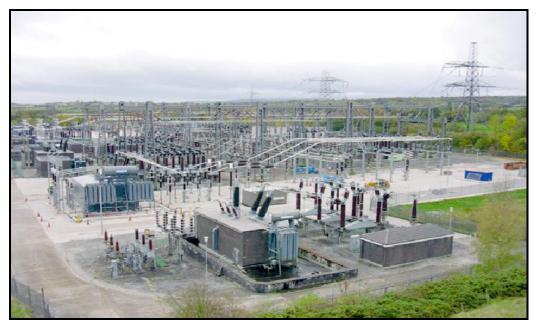
Figure 8.4: Air Insulated Substation (Source: <u>http://www.foxitsoftware.com</u>)
